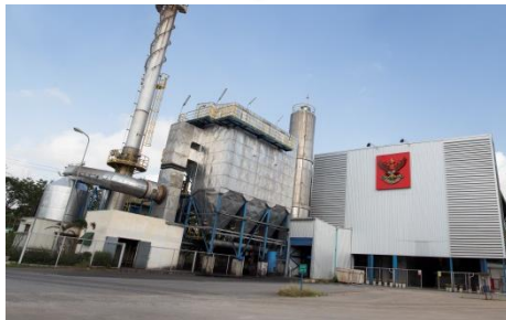
Hat Yai Waste to Energy Power Plant
