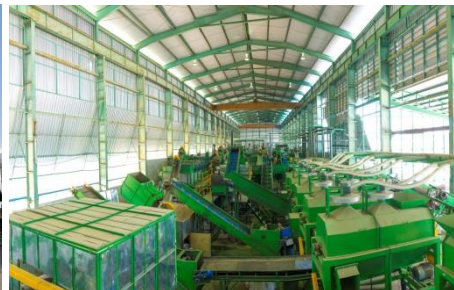
Waste Plastic Recycling Plant
