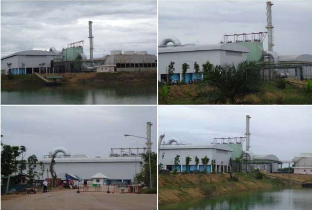
Figure 7: Biomass power plant in Sa Kaeo (SK1)
